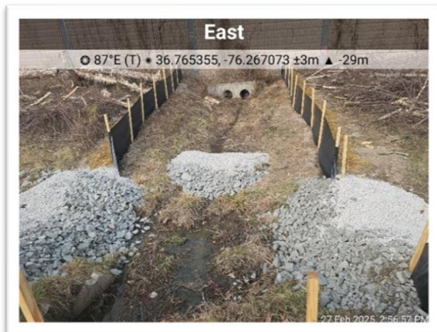
Culvert Inlet Protection and Silt Fence (Ramp A)
