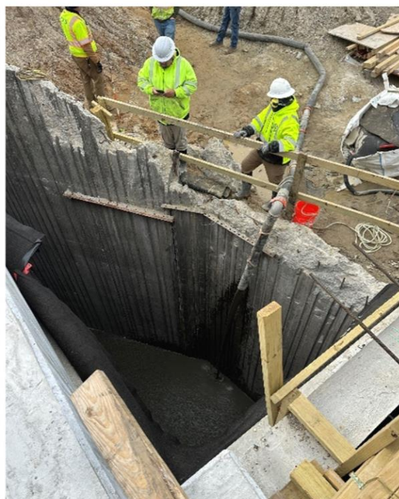
Placement of Lightweight Concrete Fill between existing wingwall and new wingwall, East Abutment for WB Hampton River Bridge
