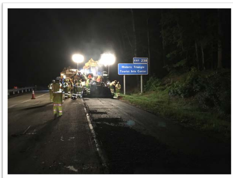
I-64 westbound outside shoulder strengthening operation
