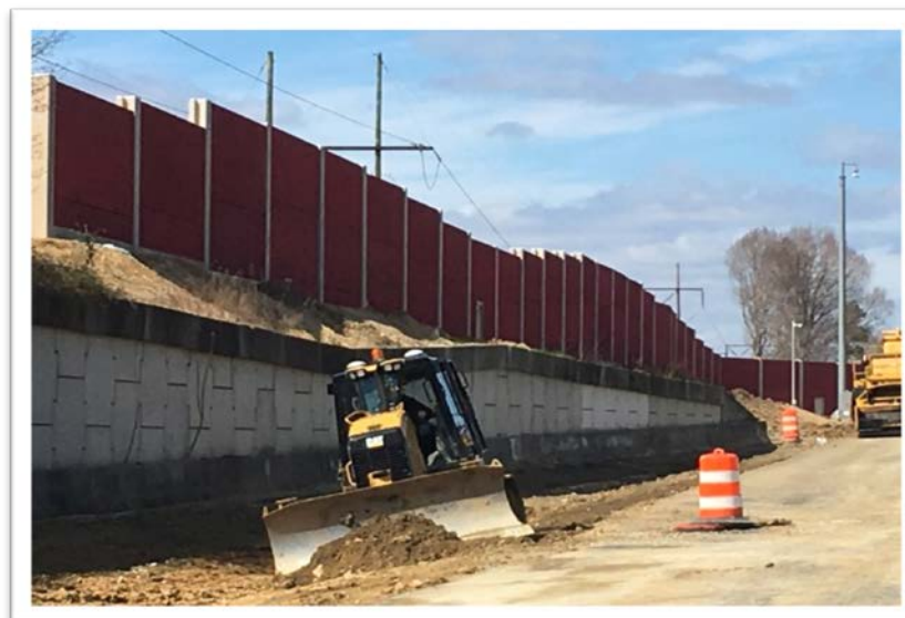
Eastbound I-64 noise wall and ditch grading
