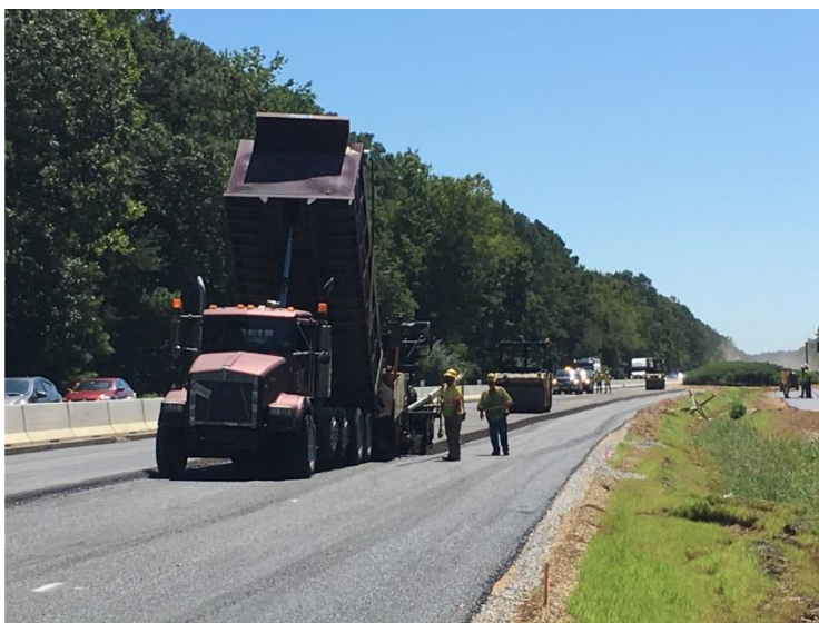
Asphalt and CCPRM placement westbound I-64 median
