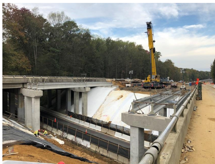
Concrete beam installation at Lakeshead Drive Bridges
