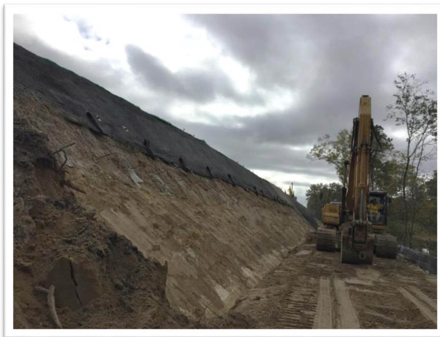
Constructing Soil Nail Wall, I-64 EB
