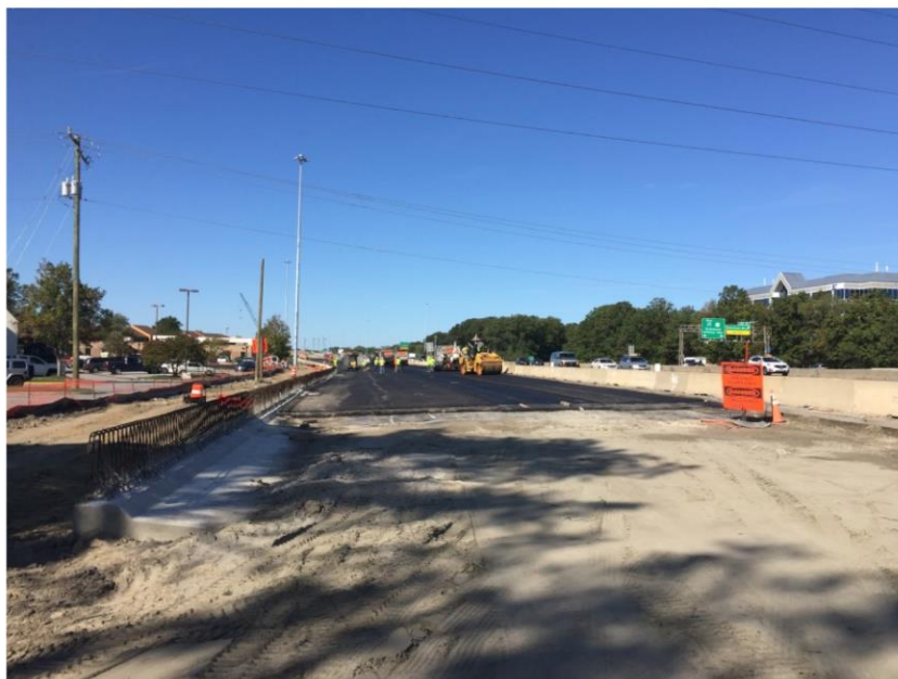
Placing Base Course, I-264 EB
