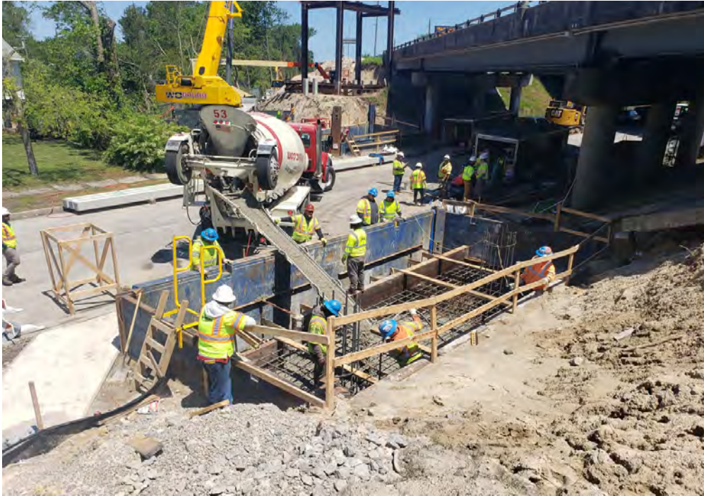
◀ Mason Creek Rd Bridge Placing concrete for Pier 2 footing for eastbound widening
