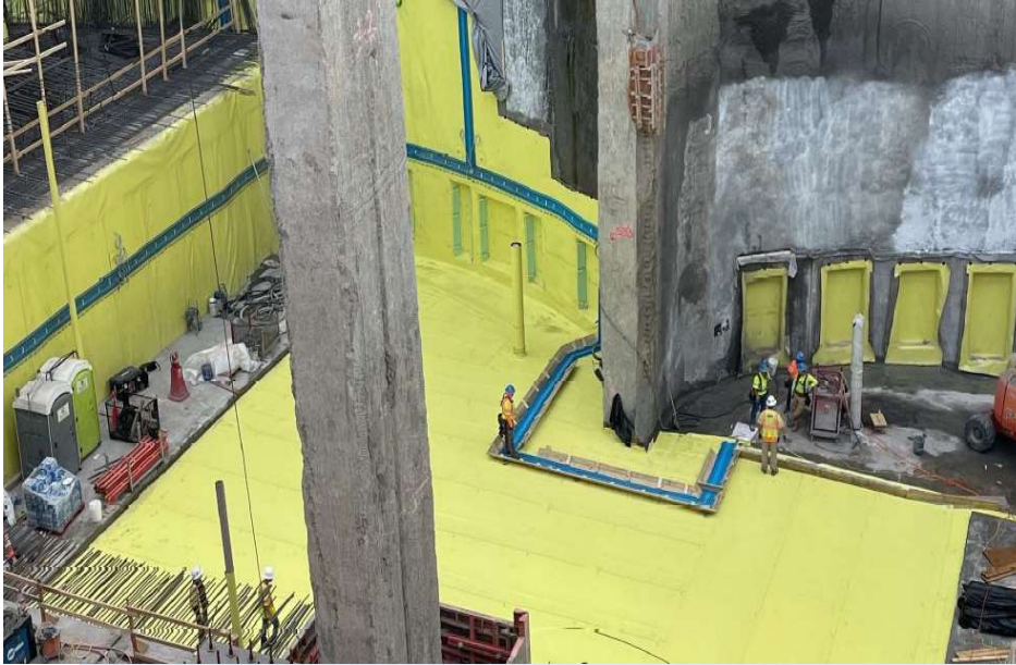
◀ South Island Waterproofing membrane installation in Cell 1 and Cell 2
