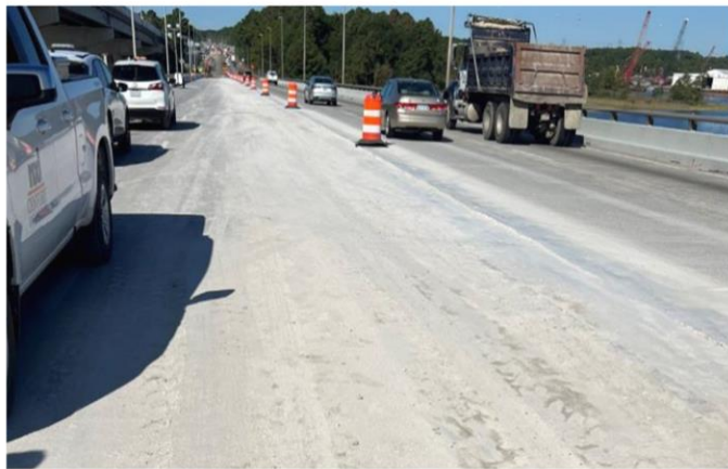
Median Barrier removed from Old High Rise Bridge (Looking West)
