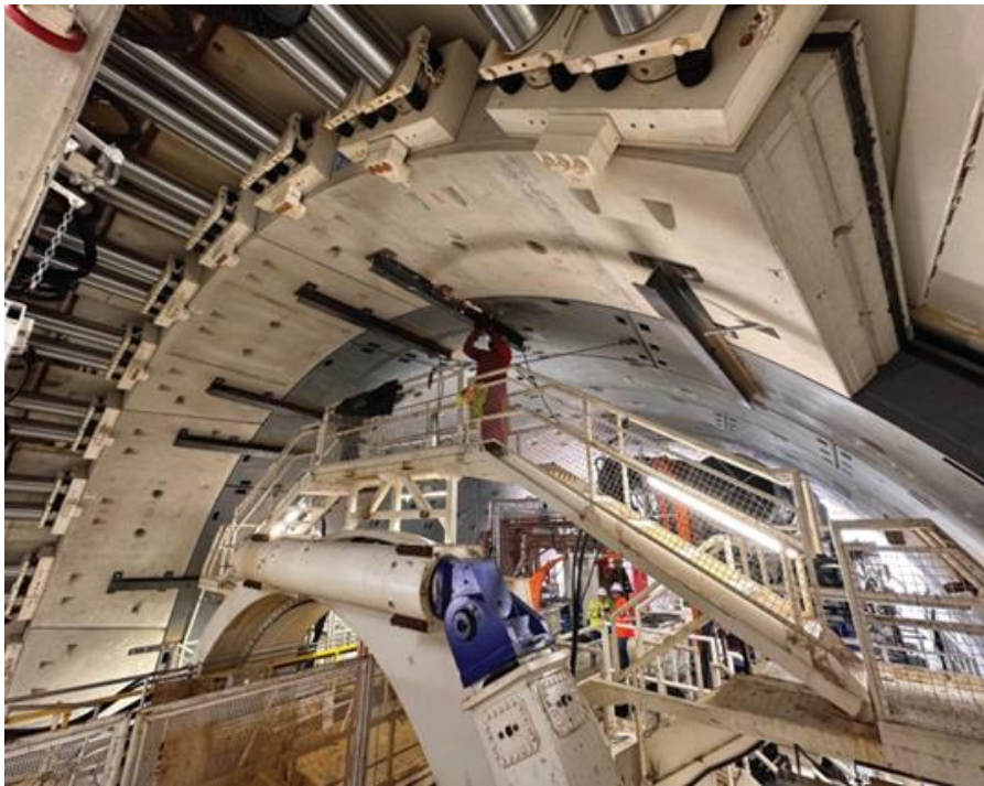
◀ HT Tunnel TBM assembling permanent ring #1
