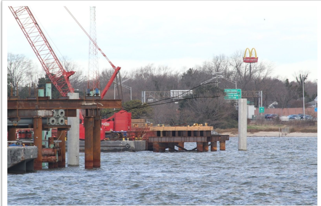
Pile Beams and Decking on Temporary N1 Construction Trestle
