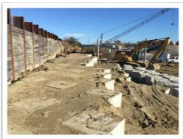
Newtown Bridge Pile Caps for Ground Improvements
