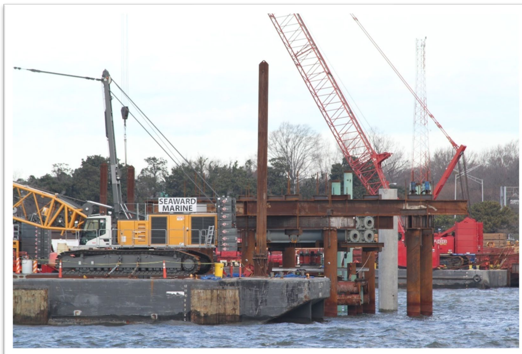
Framing for Static Load Test of 54" Cylinder Pile
