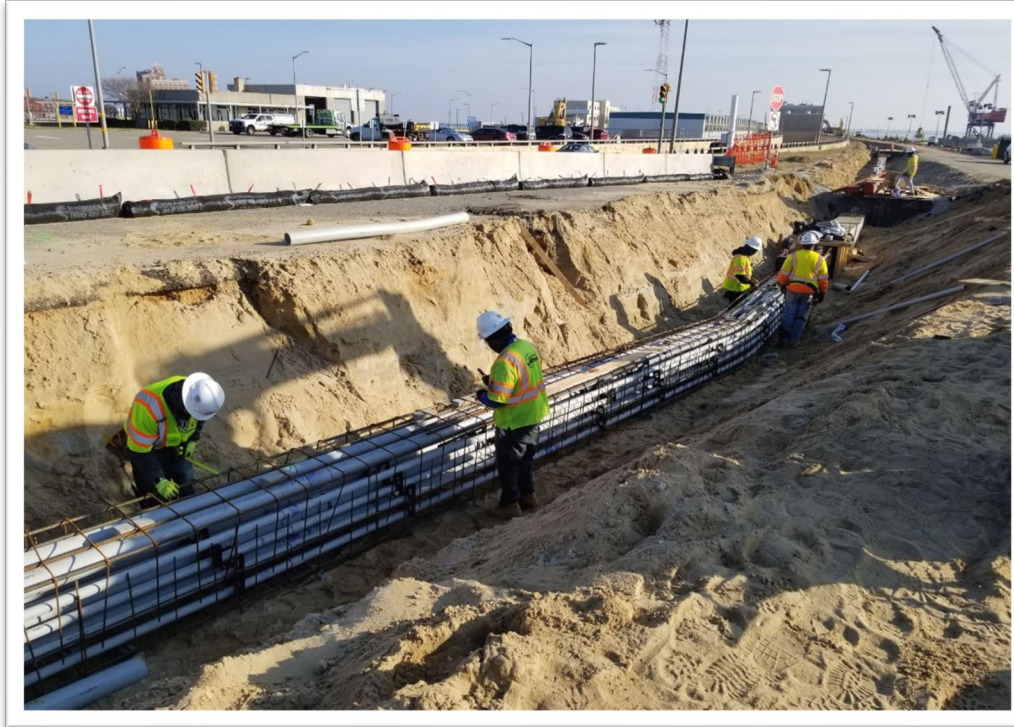
North Island Medium Voltage Duct Bank Install
