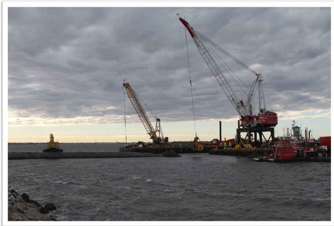
Placing Perimeter Stone for North Island Expansion
