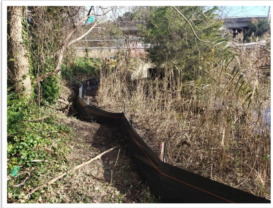
Erosion and Sediment Controls at Bay Avenue
