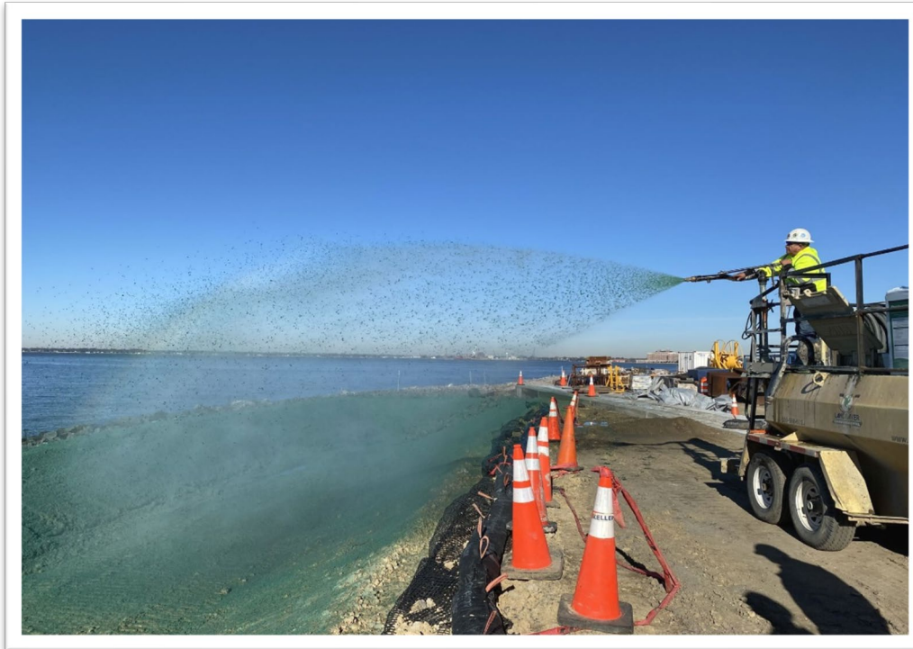
South Island Hydroseeding Completed Sediment Pond
