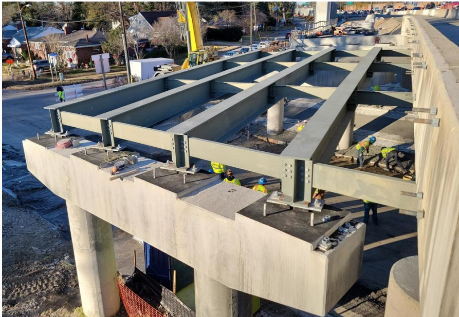
◀ Evans St. Bridge Eastbound View of Span 2 steel girders installed
