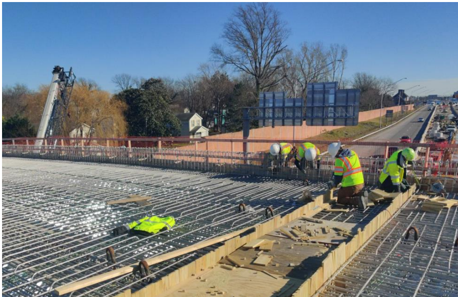
◀ Mallory St. Bridge Eastbound Installation of bridge deck reinforcing steel and formwork
