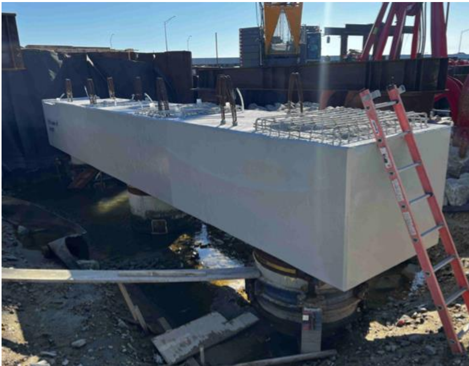
◀ South Trestle Ramp A Bent 7 cap placed
