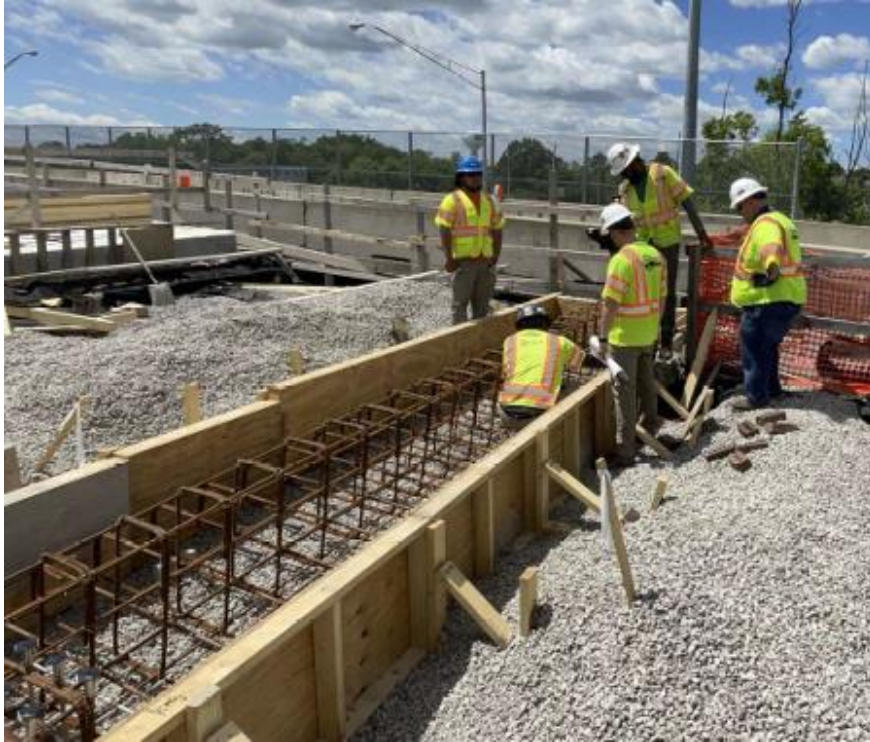
◀ Mallory Street Bridge Eastbound Approach slab work at Abutment B
