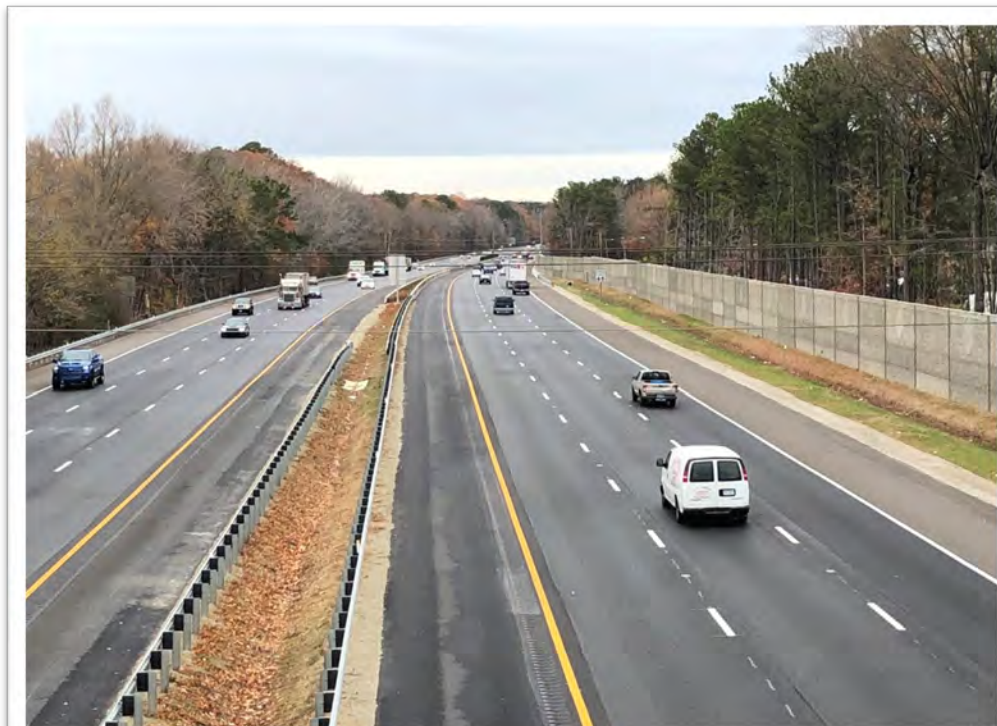
Project Site (Looking West from Denbigh)
