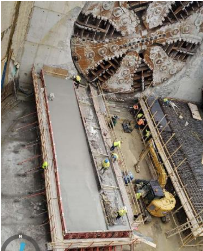
◀ North Island Concrete pour for TBM Cradle (east-side)
