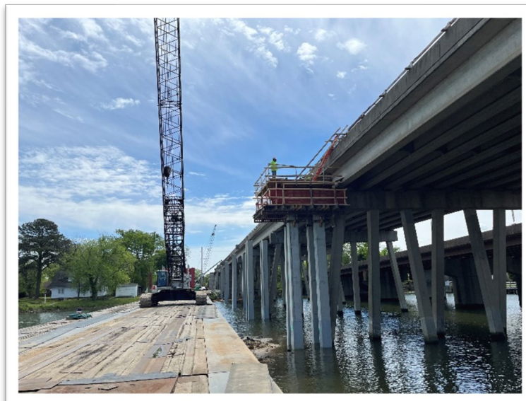
HREL 4C bridge widening work at WB I-64 over the Hampton River
