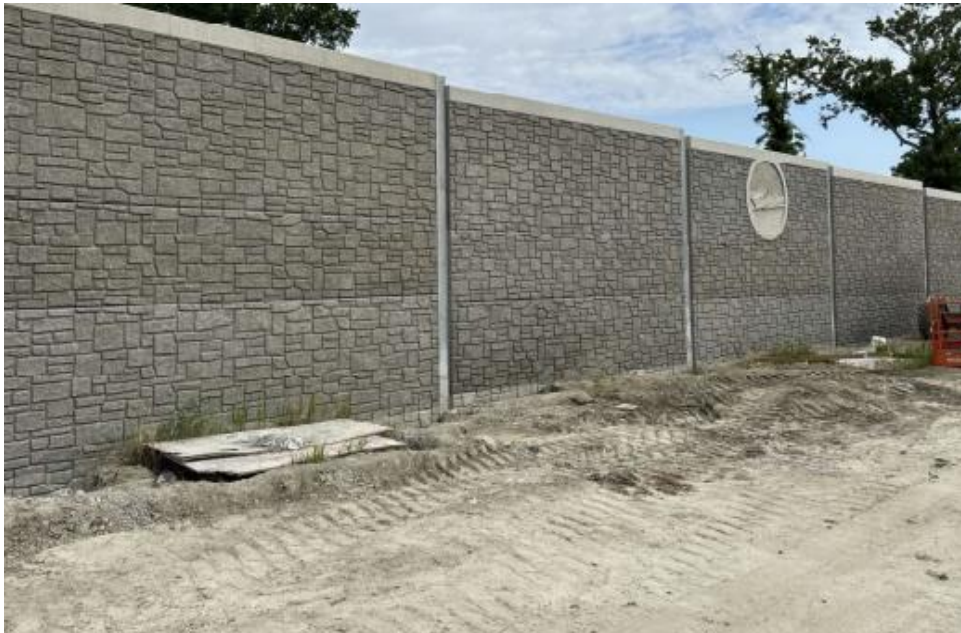
◀ I-64 near Mason Creek Road Panels installed at sound wall 4-1A.
