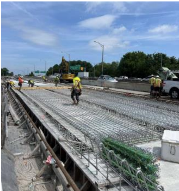
◀ Bay Avenue Bridge Eastbound Deck reinforcement installed at Spans 20 - 22
