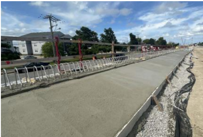
◀ Retaining Wall 302 near Bayville St. exit Moment slab placement
