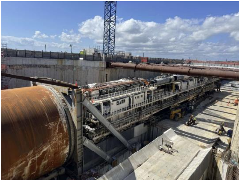
◀ GP Tunnel Gantries 1, 2, and 3 in the launching position behind the shield.
