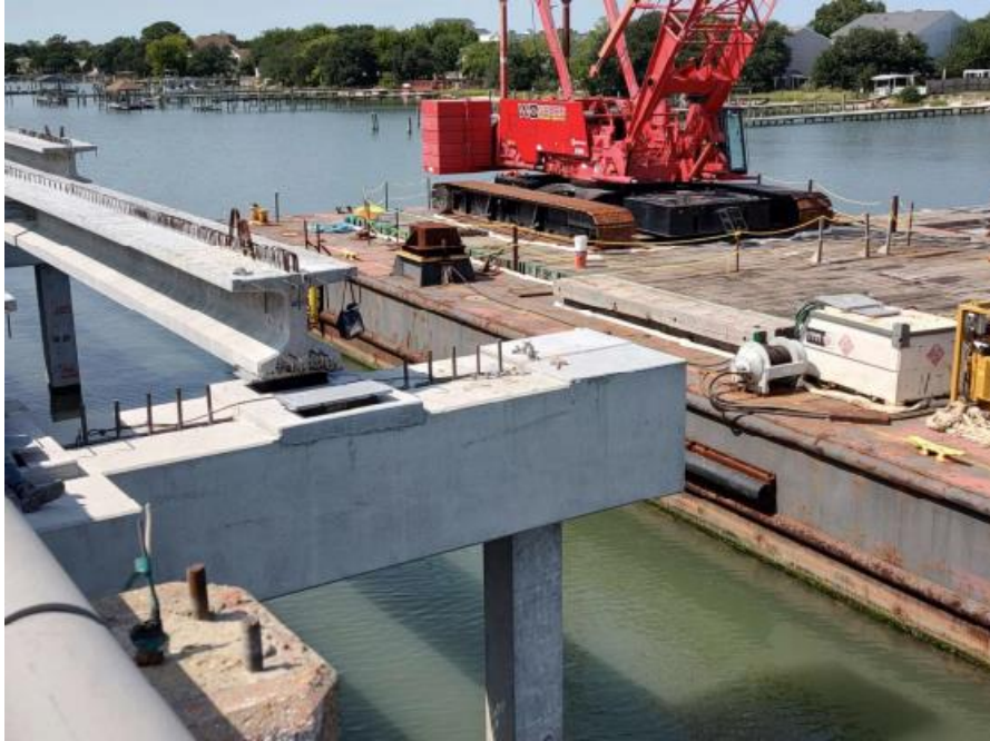
◀ Willoughby Bay Bridge Westbound Installation of girders at Bent 38
