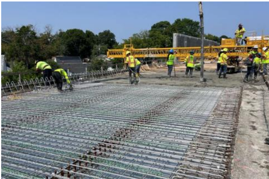
◀ Mason Creek Bridge Eastbound Deck placement for Spans 1, 2 and 3
