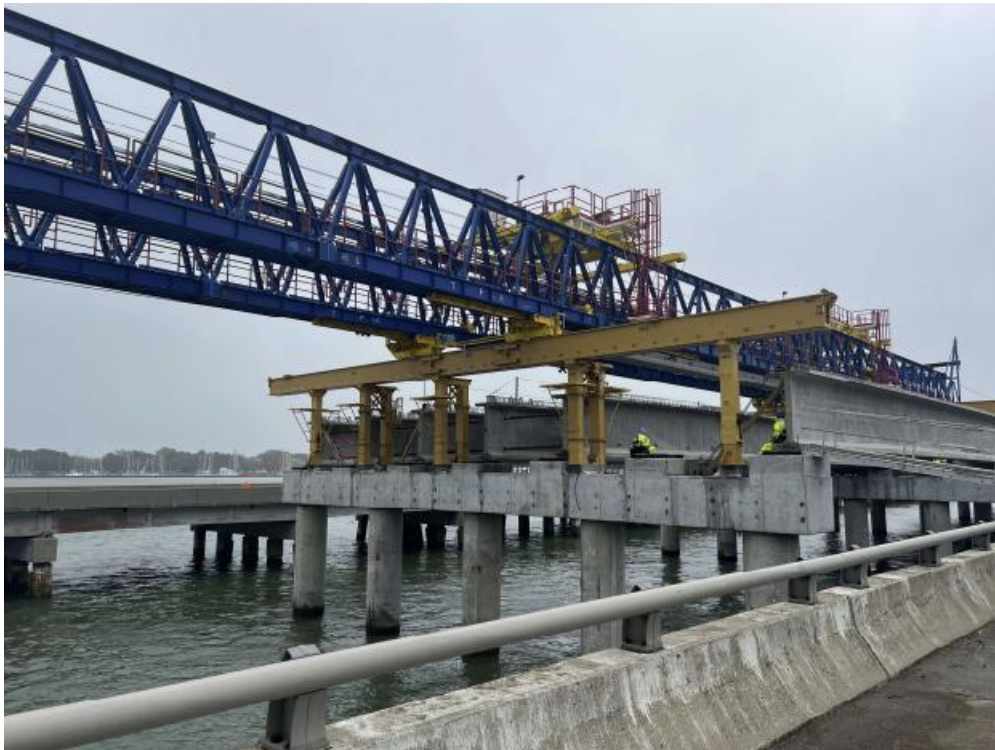
◀ North Trestle Westbound Beam Launcher installing girders at Span 21
