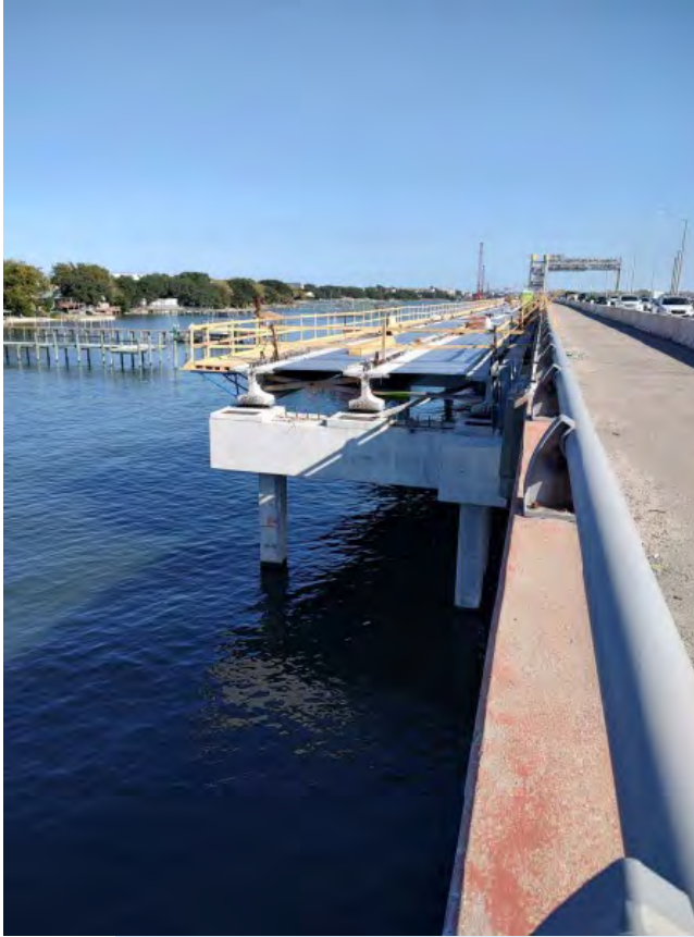
◀ Willoughby Bay Bridge Westbound Installation of OH Jacks from Bent 13 to Bent 40
