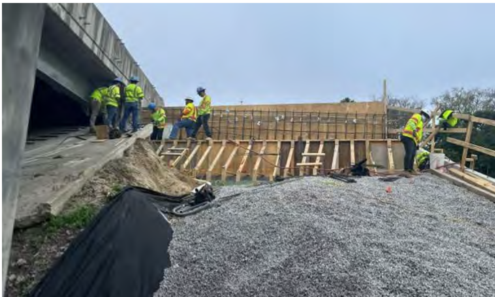
◀ Evans St. Bridge Eastbound Installation of footing and backwall at Abutment B
