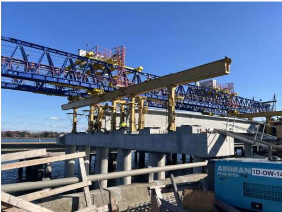
◀ North Trestle Westbound Installing Span 16 girders
