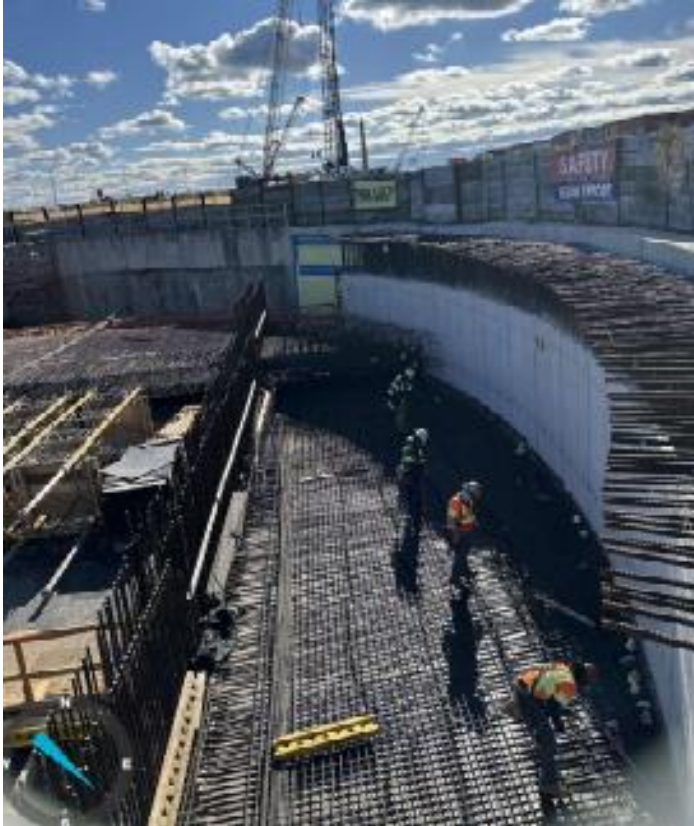
◀ South Island Rebar for plenum slab in Cell 3 east.
