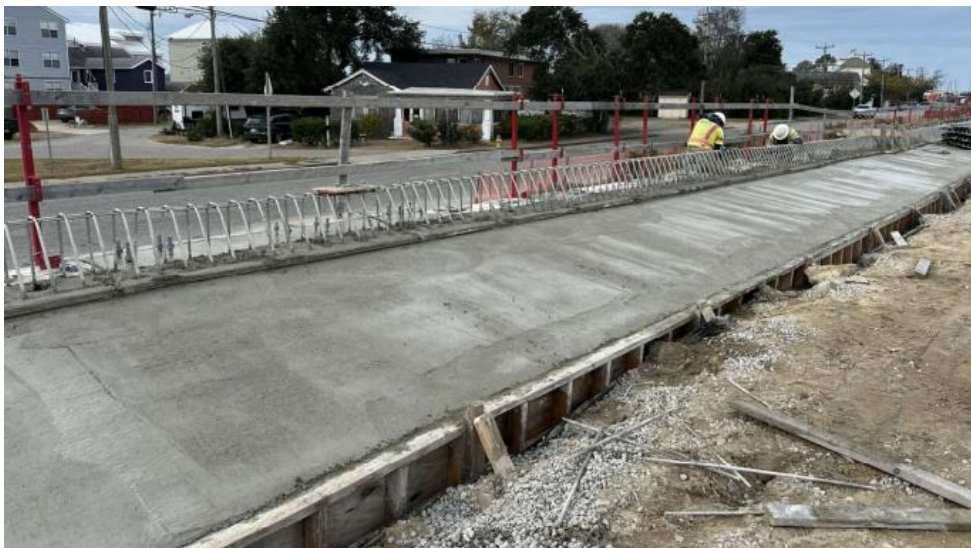
◀ Retaining Wall 302 on Bayville Street Moment slab concrete placed
