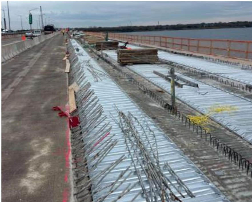
◀ Willoughby Bay Bridge Eastbound Stay-in-Place (SIP) installation
