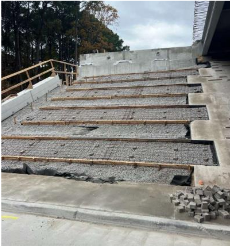
◀ Patrol Road Bridge Eastbound Abutment A slope protection
