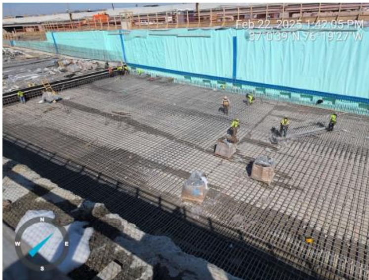
◀ North Island Rectilinear Approach Base Slab Pour 4 Reinforcing Steel
