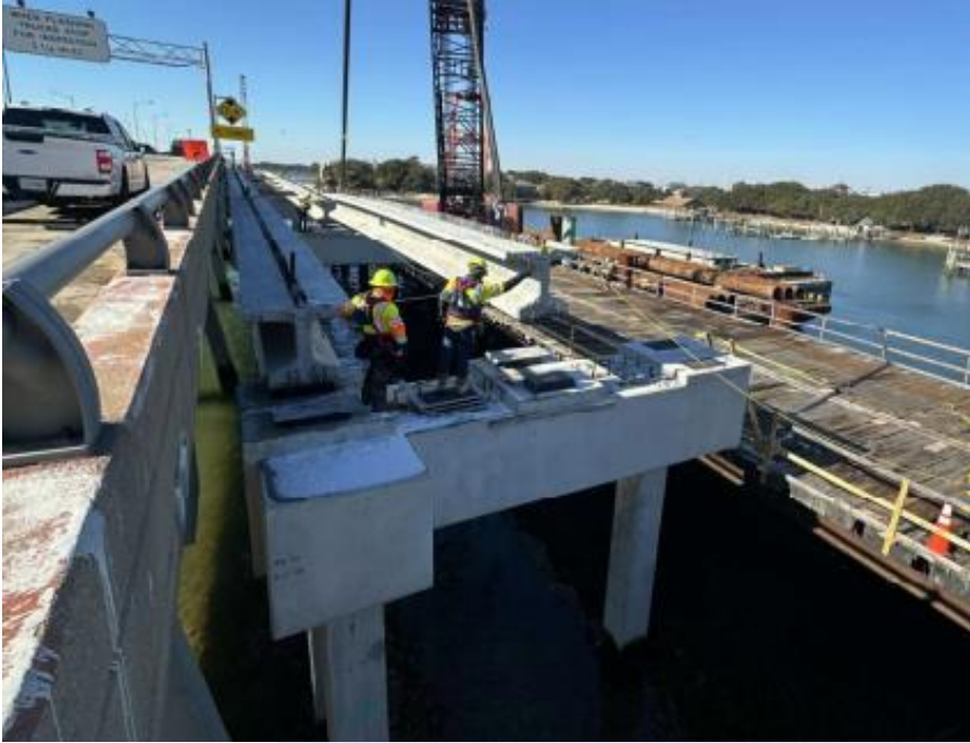
◀ Willoughby Bay Bridge Westbound Setting girders at Span 71
