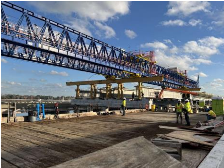
◀ North Trestle Westbound Installing Span 14 girders
