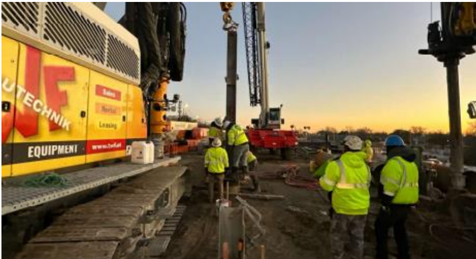
◀ Retaining Wall 309 near 4 th View St. Columns continue to be installed
