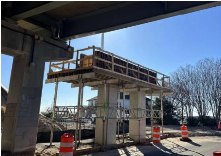
◀ 13 th View St. Bridge Eastbound Pier 2 cap installation
