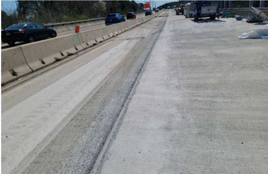
◀ Oastes Creek Type A Milling at the Phase Line
