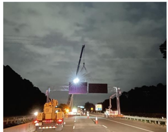
Overhead Sign Structure Installation
