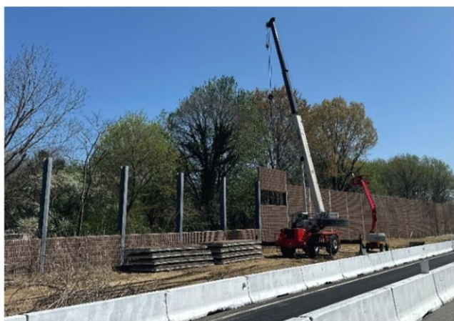
Ramp A Noise Wall Demolition
