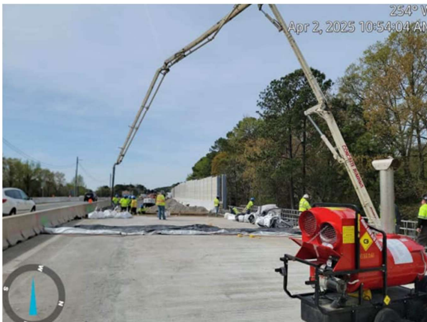
◀ Bayview Bridge Approach slab abutment B placement
