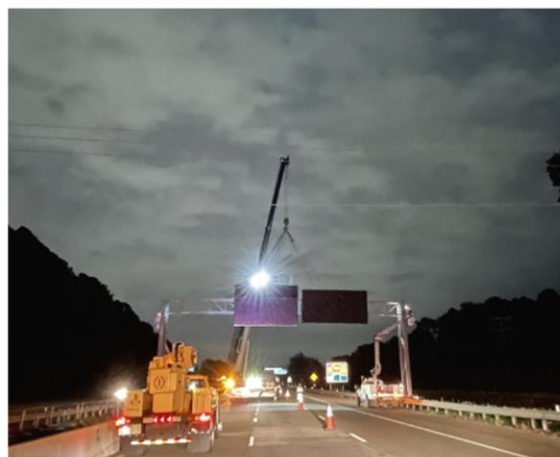
Overhead Sign Structure Installation
