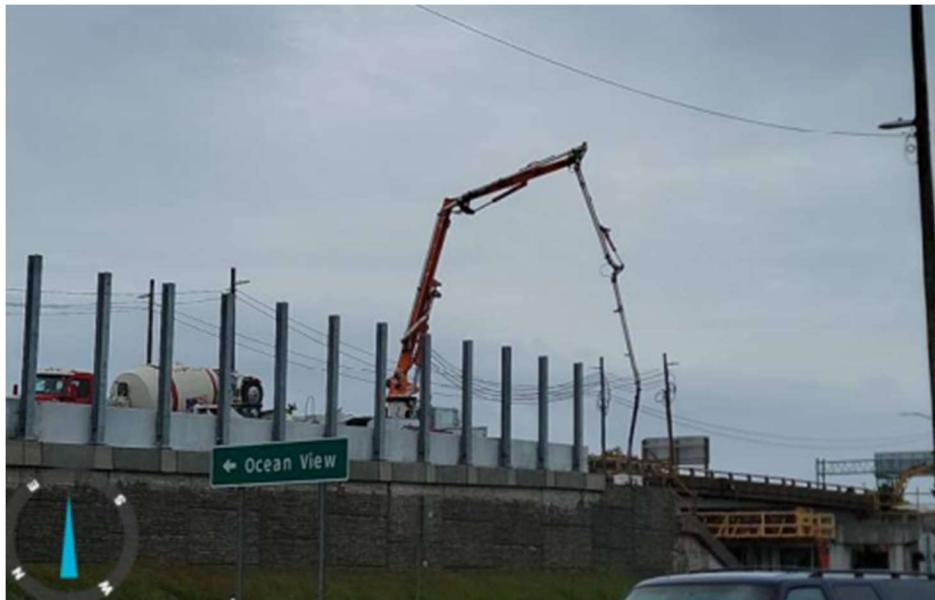
◀ 13 th View Pier 1 cap placement eastbound
