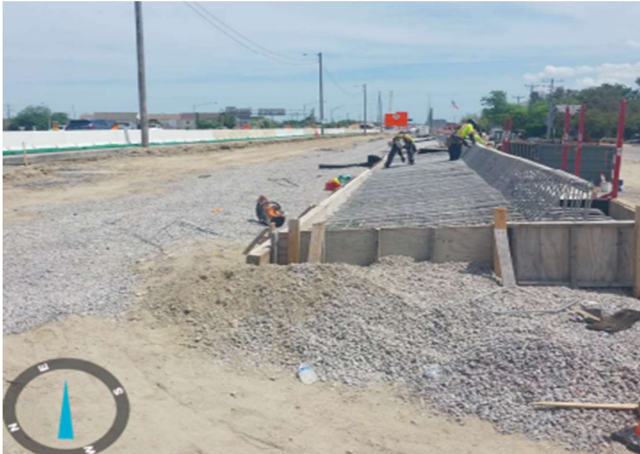
◀ Segment 3 Retaining Wall 302 moment slab work
