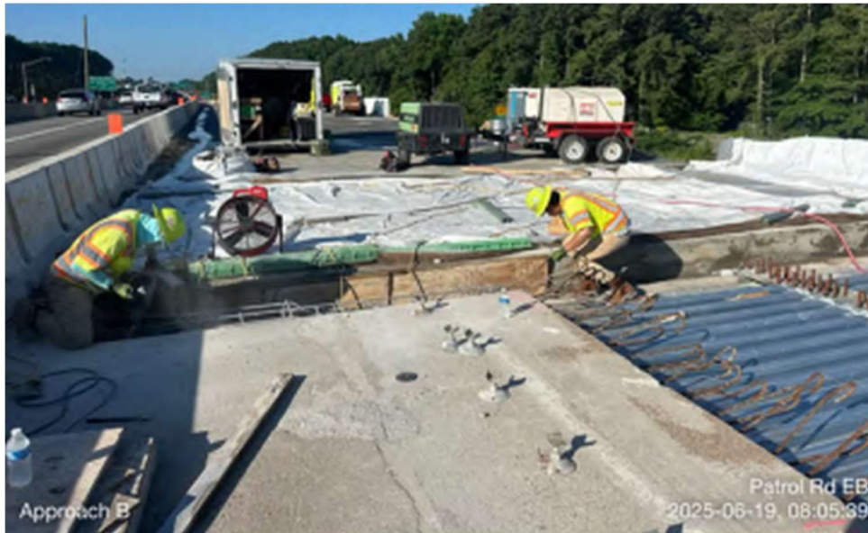
◀ Patrol Rd. (EB) Approach Slab B Placement
