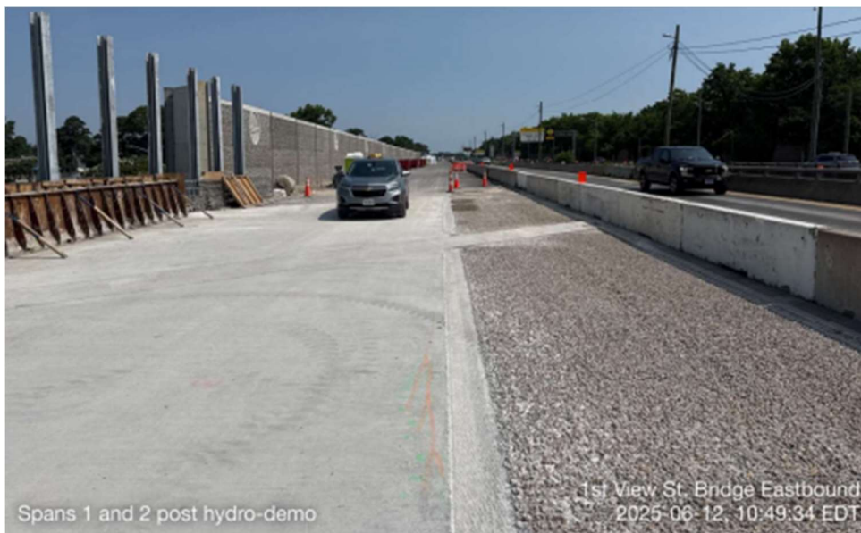
◀ 1 st View Bridge Hydro demolition Type A performed
