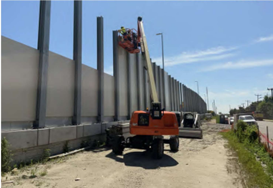
◀ Segment 3B Soundwall Panel Installation along Bayville St.
