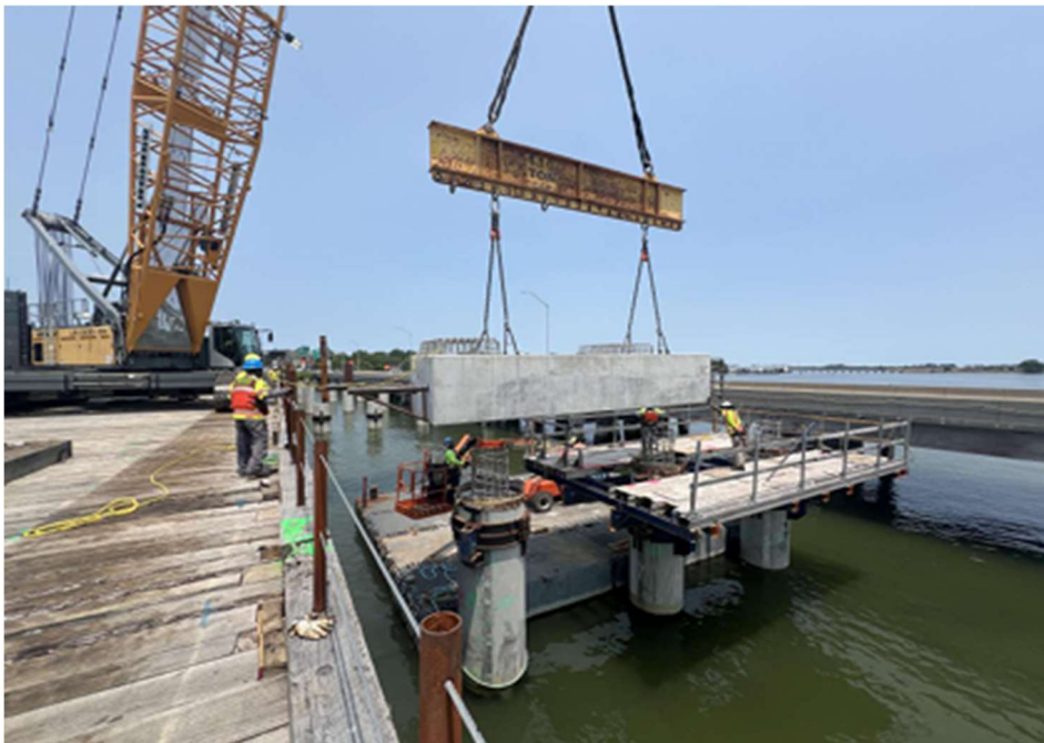
◀ North Trestle Westbound Bent 8 Cap Installation
