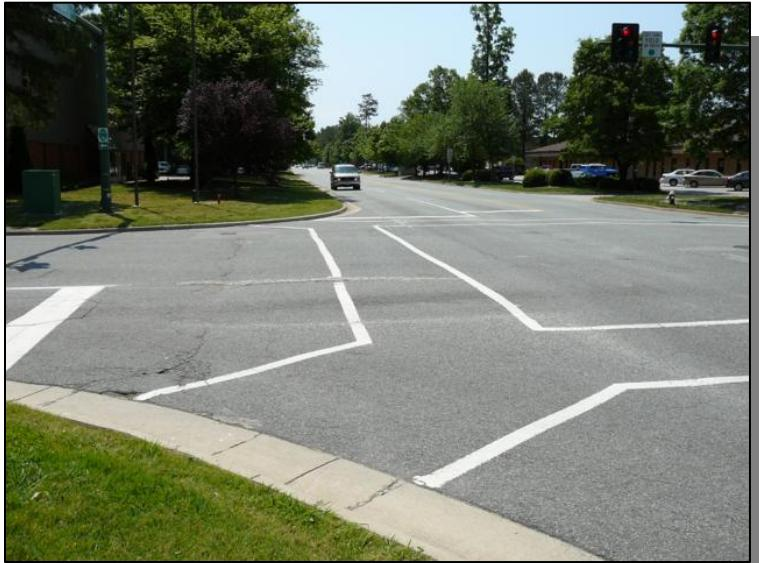
*Curb ramps and sidewalks are needed surrounding the intersection of Middle Ground Blvd and Canon Blvd.*
