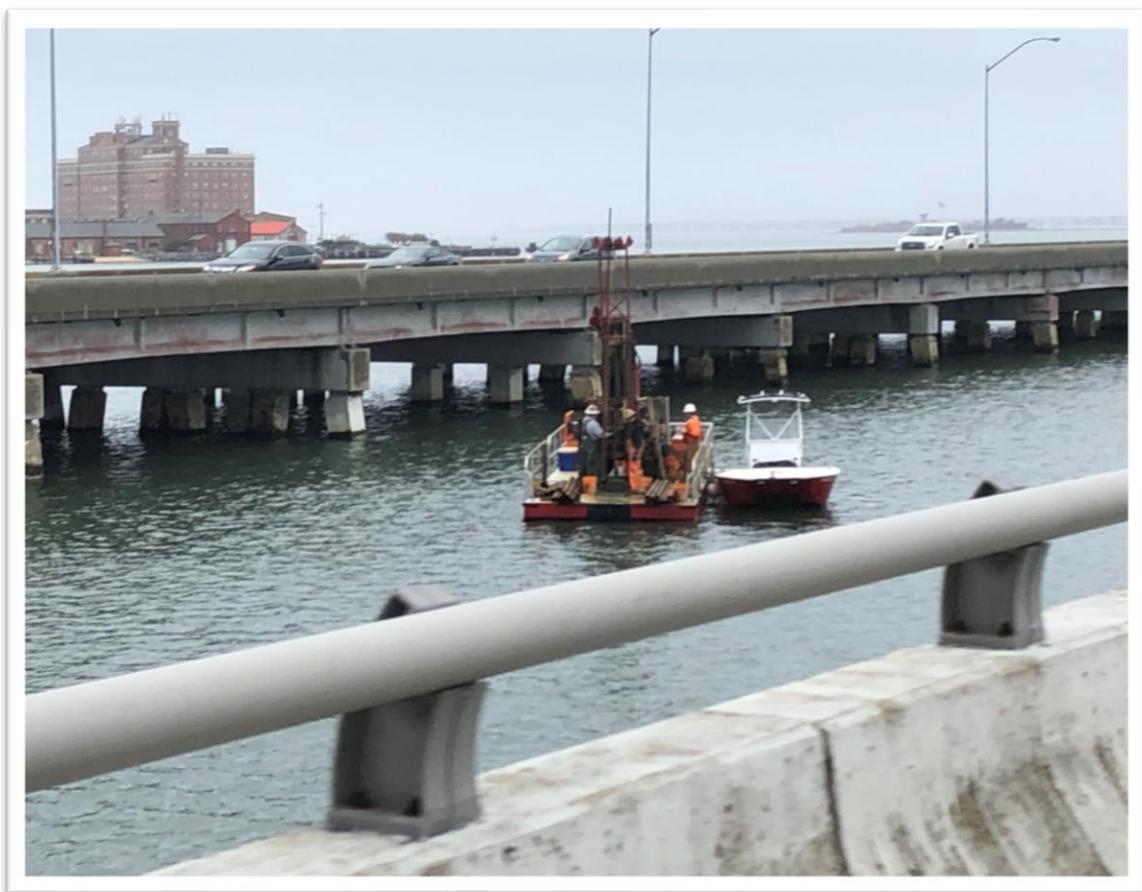
Marine Geotechnical Boring
