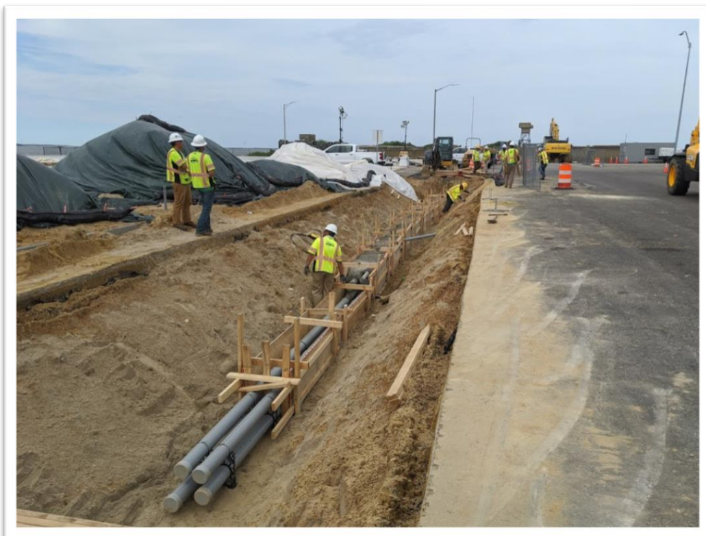
Temporary Electrical Ductbank Installation
