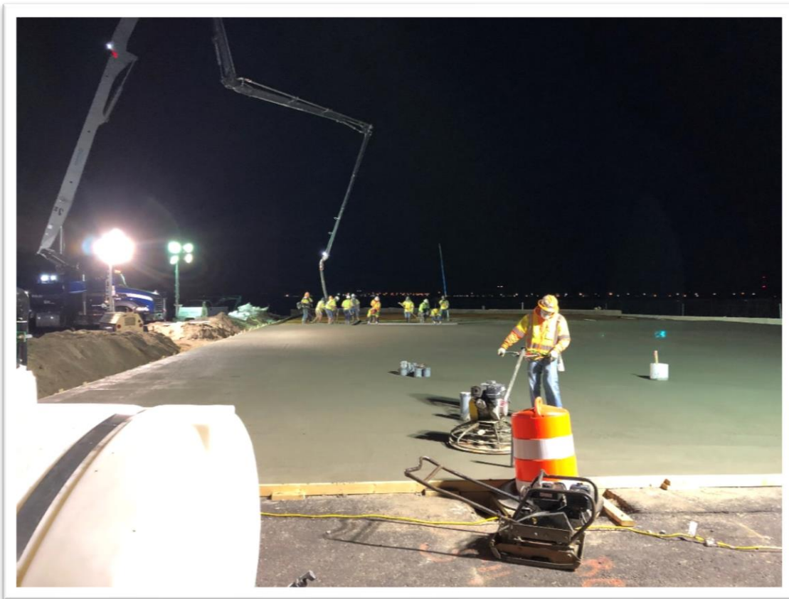
South Island Temporary Facilities Slab Foundation
