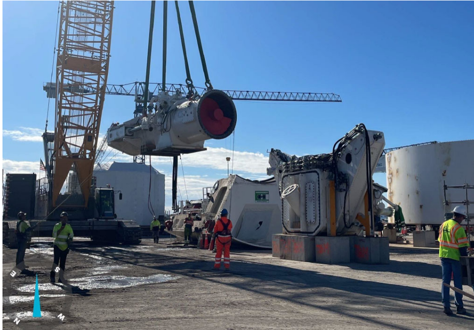
◀ South Island Assembly of TBM components (screw conveyor and crusher box)
