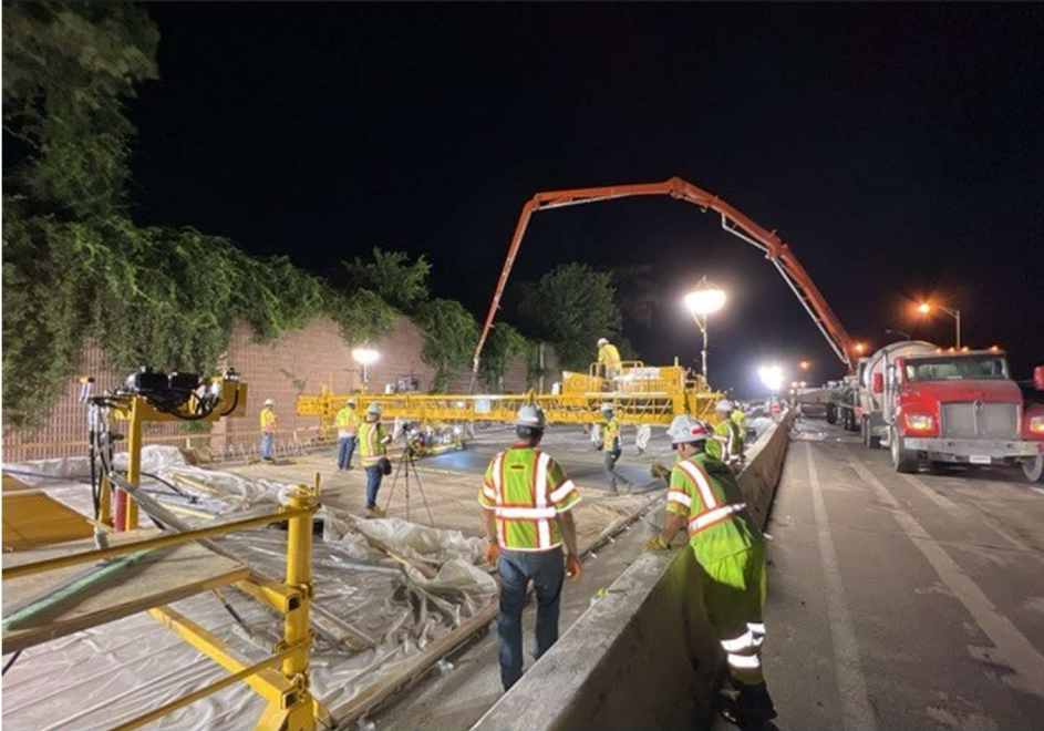
◀ Bay Avenue Bridge Concrete placement for Span 27 eastbound
