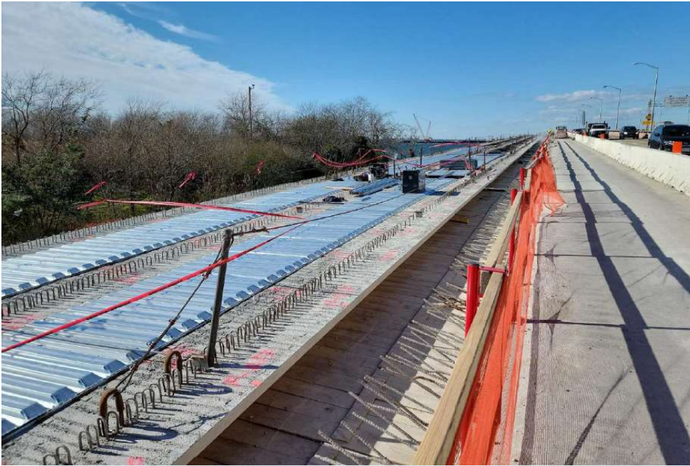
◀ Willoughby Bay Bridge Placing deck forms
