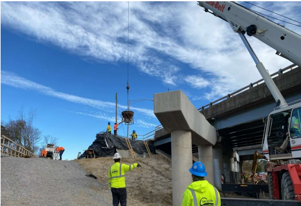
◀ Mason Creek Bridge Placing Abutment A pedestal concrete
