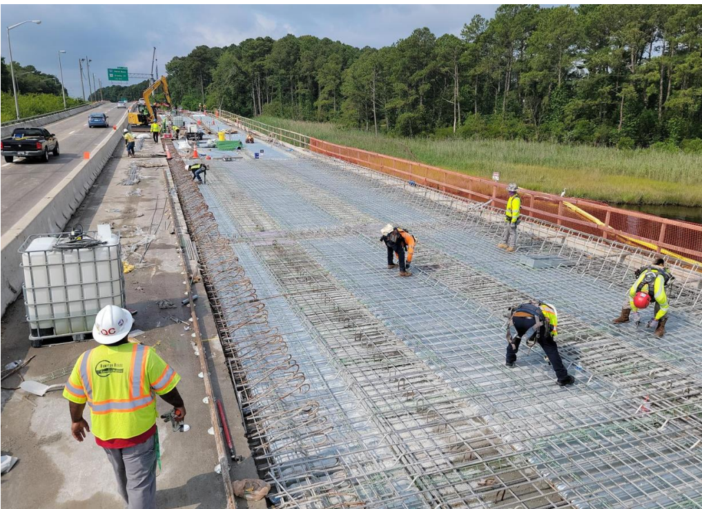
◀ Oastes Creek Bridge Eastbound Installation of bridge deck reinforcing steel
