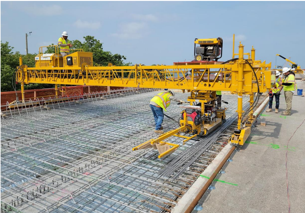
◀ Willoughby Bay Bridge Eastbound Performing dry run of screed machine for finishing concrete prior to placement of bridge deck
