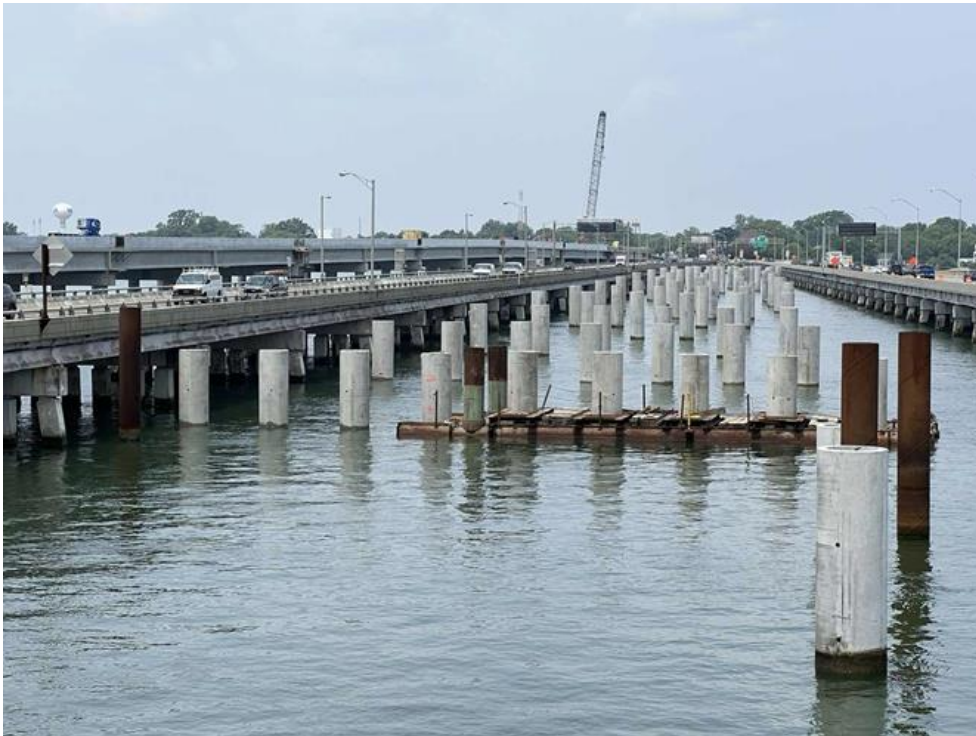
◀ North Trestle Westbound Completed Bent 26 pile group
