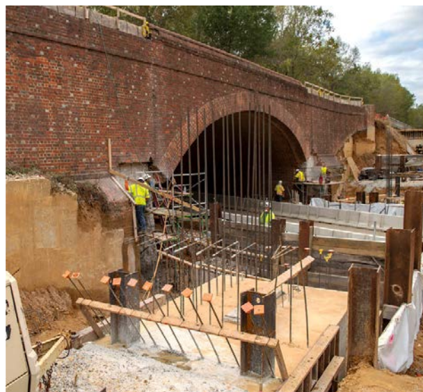
Bridge widening and brick masonry work along I-64 over Colonial Parkway
