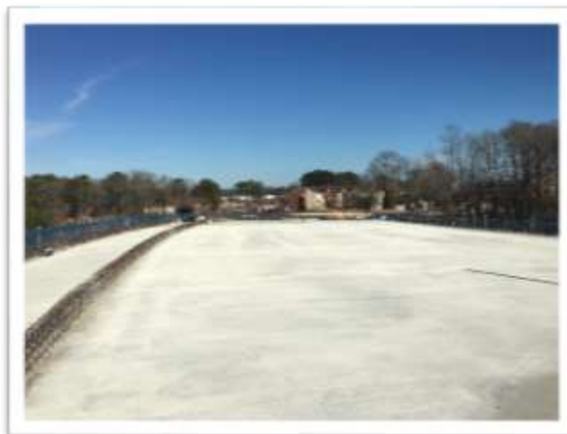
Five of Seven Deck Sections Placed - Flyover Bridge (B603)
