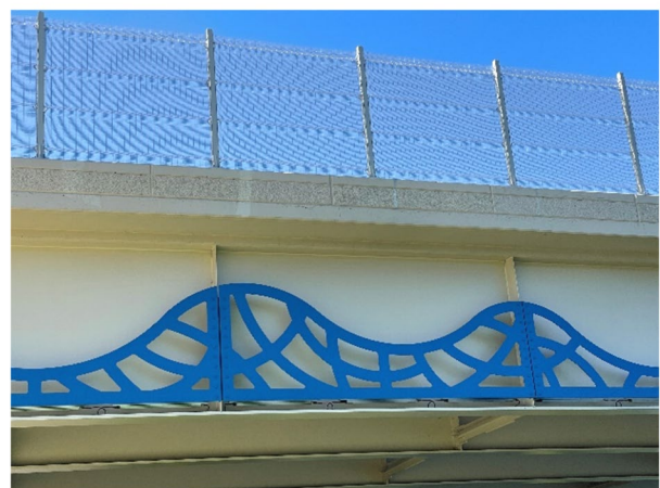
Flyover Bridge with Pedestrian Fence and Wave Panels
