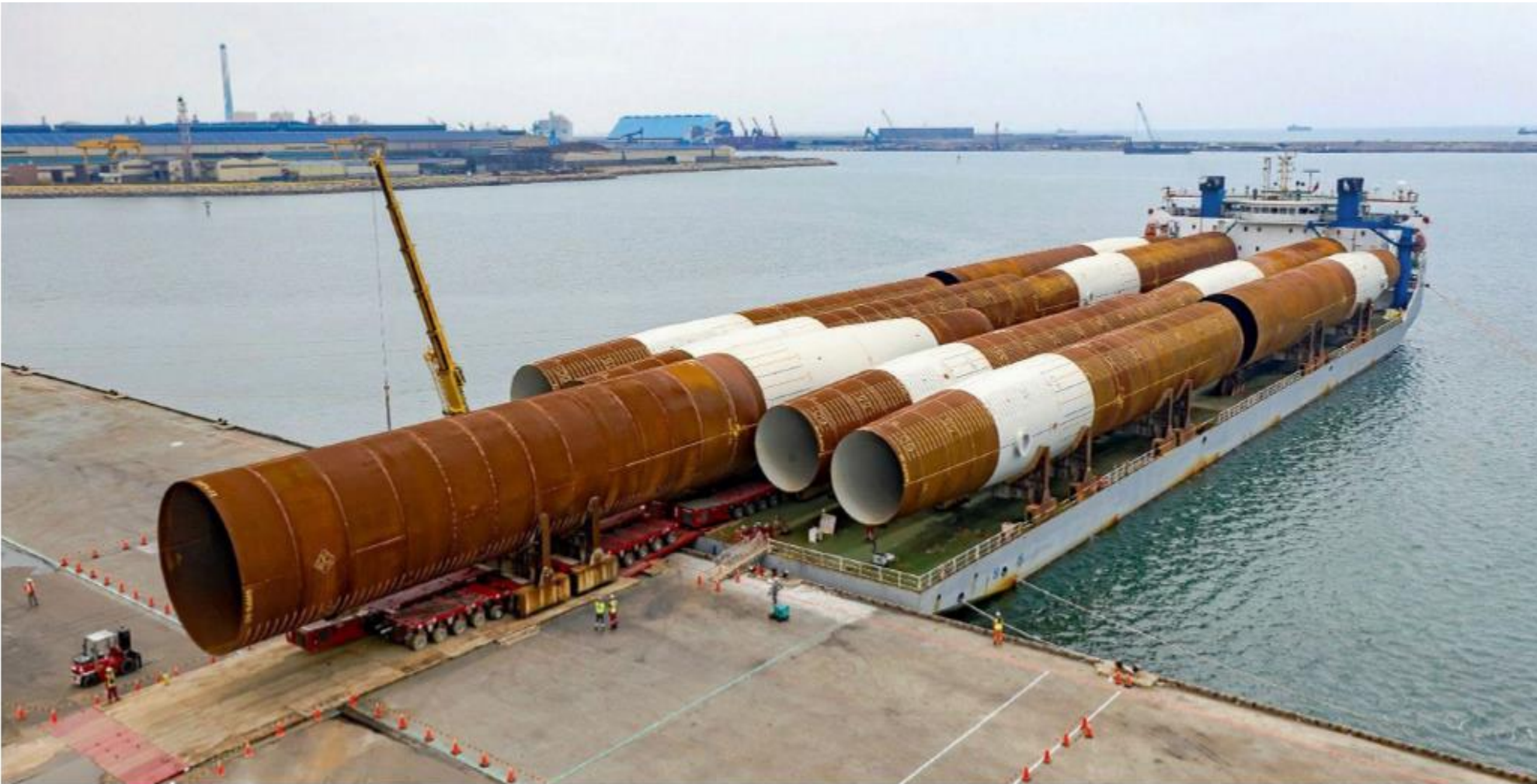
EEW SPC, Monopile load-out for Taiwanese Formosa 1 project in Rostock (GER)
