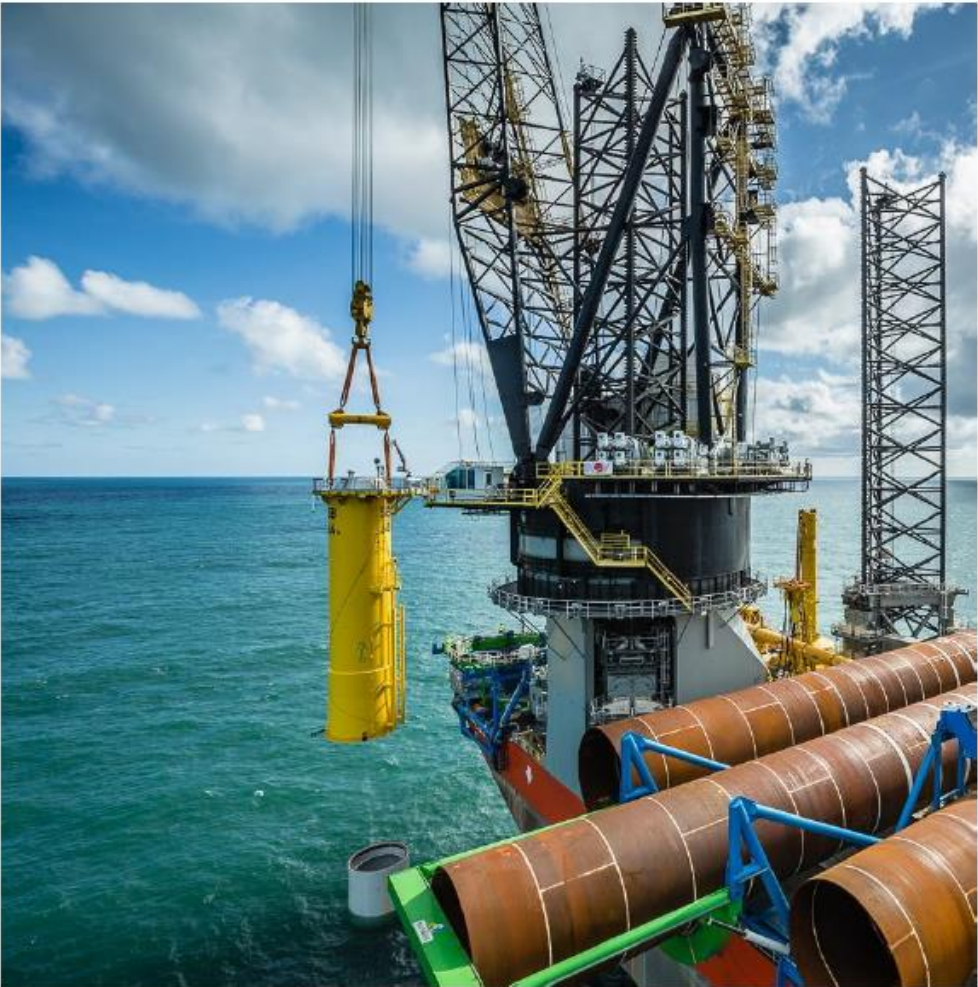
TP lift at Sandbank OWF (GER)
