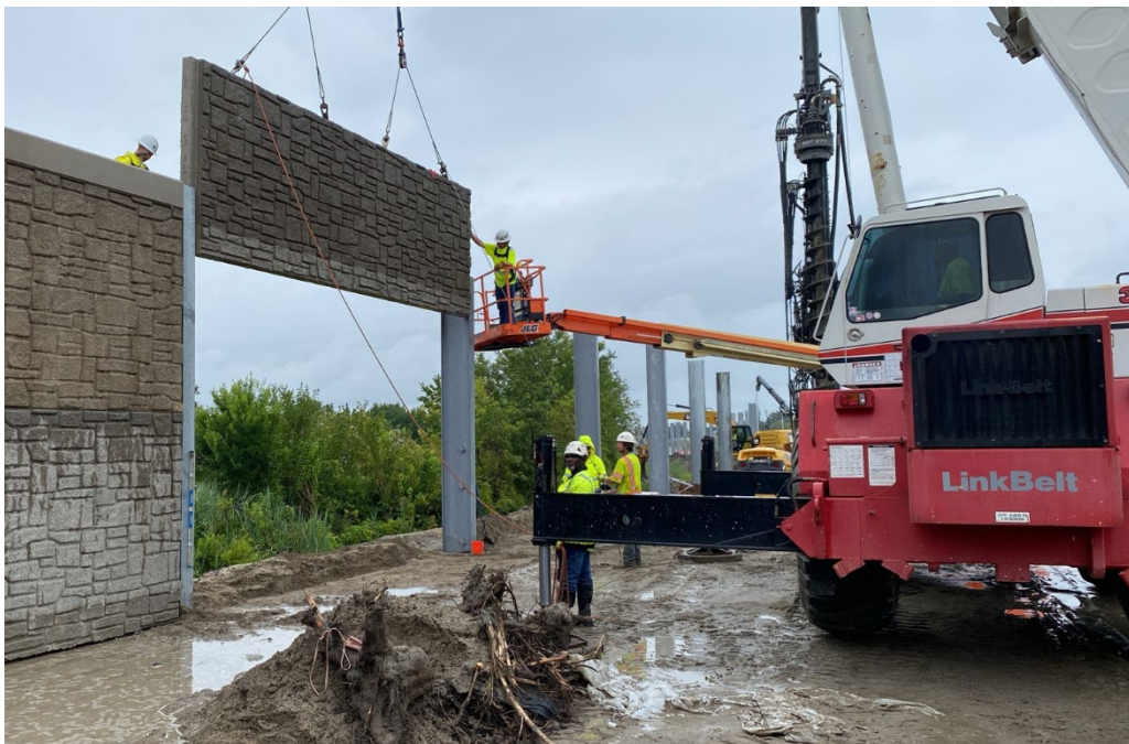
◀ Sound Wall 3-3 Panel installation on I-64 between 4 th View St. and Mason Creek Rd.
