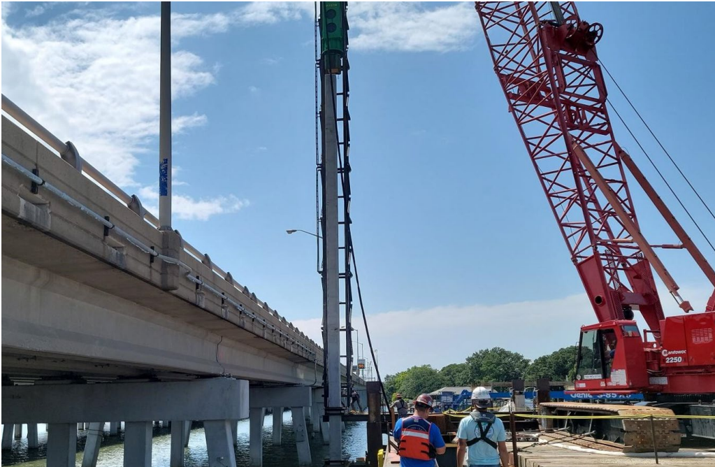
◀ Willoughby Bay Bridge Westbound Pile driving at Bent 16
