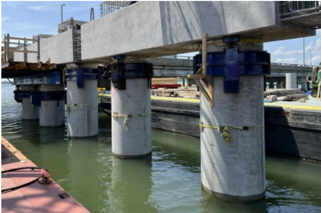
◀ North Trestle Westbound Placement of partial precast cap onto foundation piles
