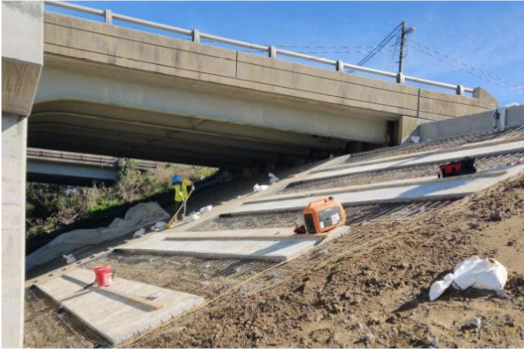
◀ 4th View St. Bridge Concrete slope protection work
