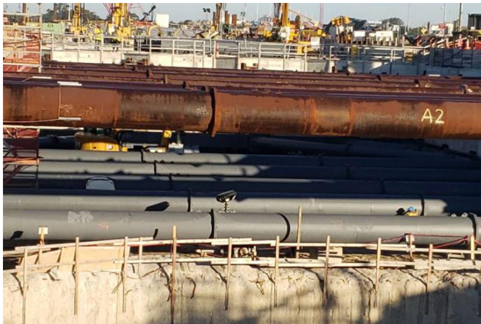
◀ North Island Installing temporary struts in Cell 2
