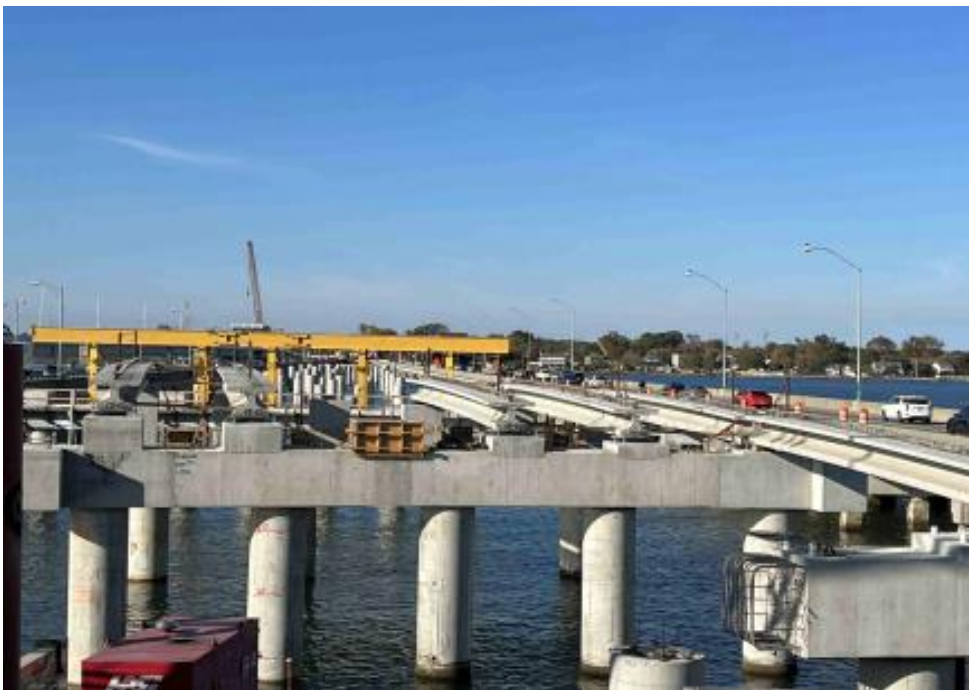
◀ North Trestle Westbound Span 1 beam erection
