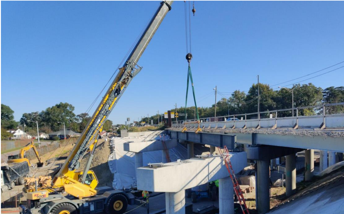
◀ 1 st View St. Bridge Setting steel girder for Span B
