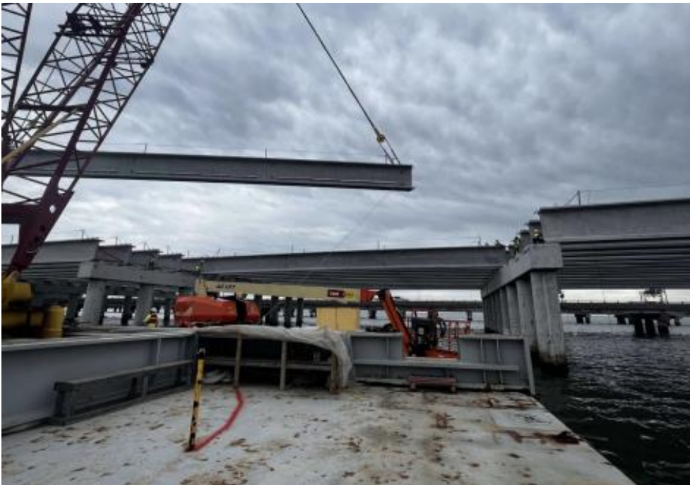
◀ South Trestle Eastbound Placement of girders at Span 20
