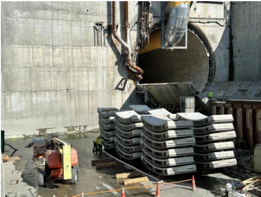
◀ HT Tunnel Segment storage in Cell 1
