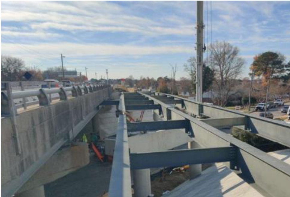
◀ Mason Creek Bridge Eastbound Girder erection
