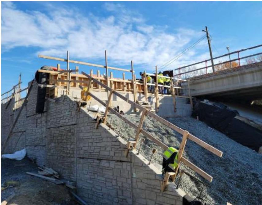
◀ Oastes Creek Bridge Eastbound Installation of backwall of Abutment A
