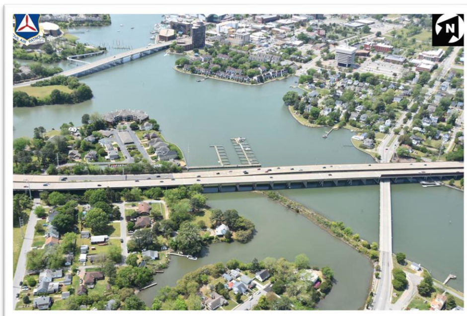
HREL 4C Hampton River Bridges
