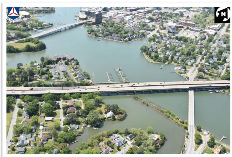
HREL 4C Hampton River Bridges
