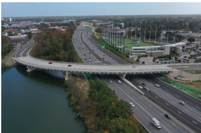
I-264 EB at Cleveland Street Flyover
