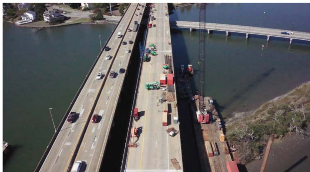
HREL 4C installation of temporary trestle along the WB 64 Hampton River bridge
