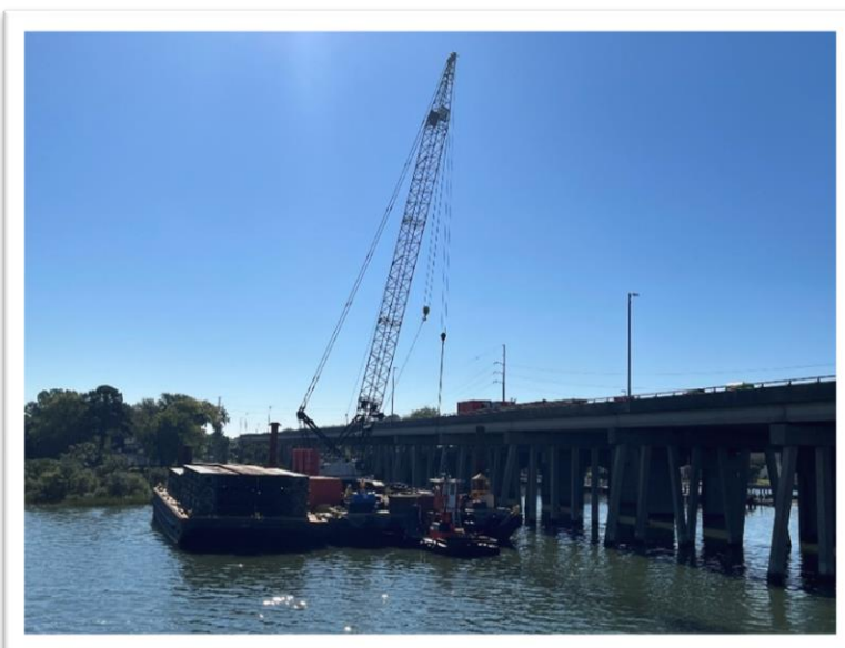
HREL 4C installation of temporary trestle along the WB 64 Hampton River bridge
