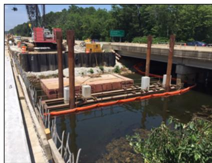
*Orange turbidity curtains, like the one pictured here, are placed around construction zones to contain sediment and protect water quality.*
